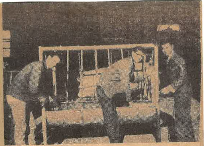
BUILDING FEEDER —Fourth year vocational agricultural students at Bellevue High School are shown above as they construct a combination hay-grain feeder in the Bellevue agriculture shop. Left to right they are Jimmy Gamblin, Charles Wells and Rick Jackson. The youths joined others throughout the nation last week in the observance of National Future Farmers of America Week.
