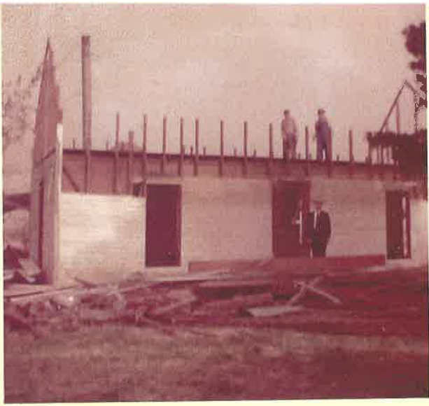
TEARING DOWN old house on Bob Reed's FARM
