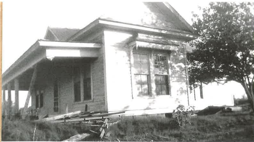
J. W. HORTON HOME BEING RE Remodded
