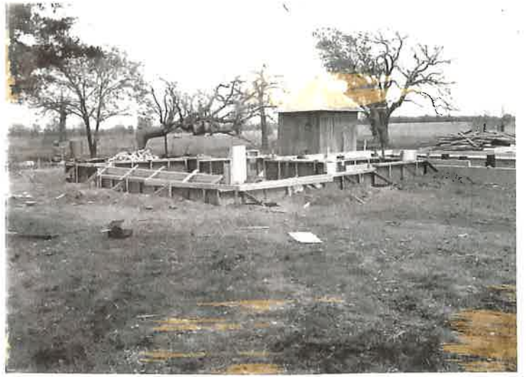
CONSTRUCTION UNDER WAY
