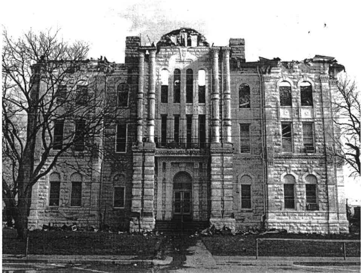
Hill County Courthouse after New Year's Day fire, 1993. (photo from THC files)
