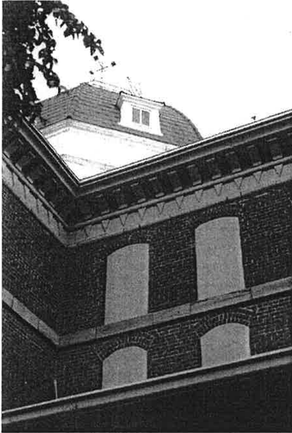
Windows that have been completely enclosed should be restored. (Photo from THC files)
