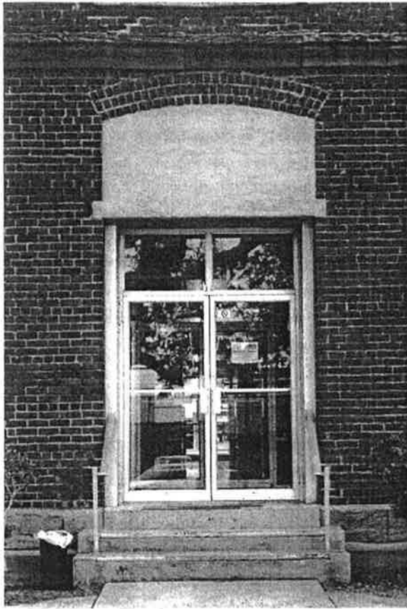
Aluminum replacement doors detract significantly from the appearance of the building. (Photo fro THC files)
