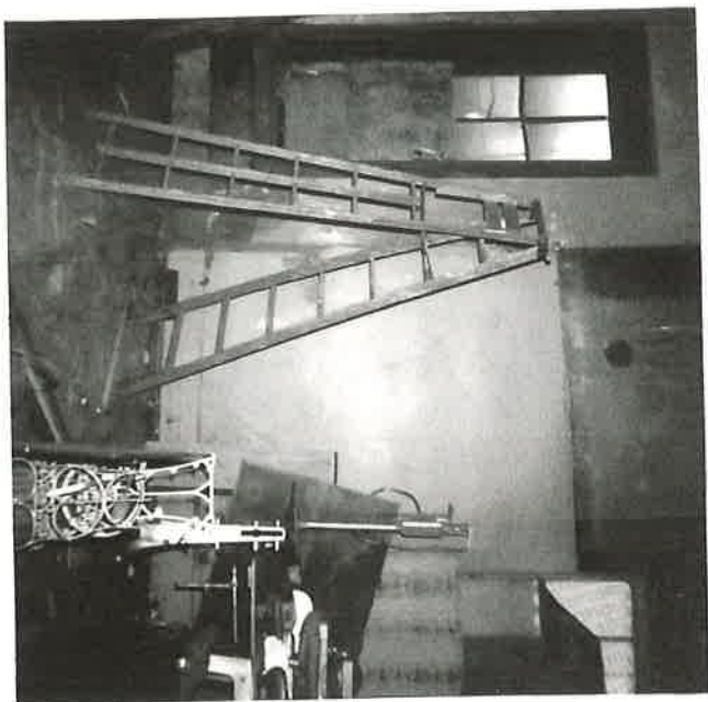
Inside Views of Building Before Remodeling Began
